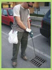
The use of tablets to treat the catch basins protected by a grill, can be improved by a tube to avoid the tablets bouncing back along the way. In fact, usually around 1/3 of the tablets don't fall into the basin, forcing us to waste time to collect
