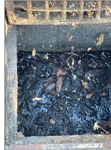
The photo shows how the uniform distribution of the vegetal oil, as well as silicon products, on the water surface depends on the presence of debris in the catch basin.
